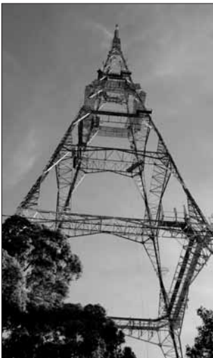
Transmission tower at Artarmon
